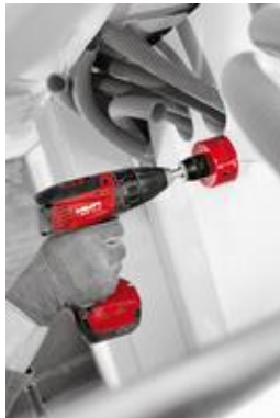
機電安裝 Electrical installation
