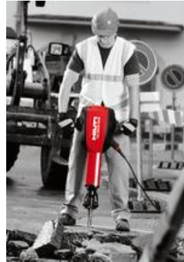
土木 Civil engineering
