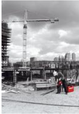
營造 building construction
